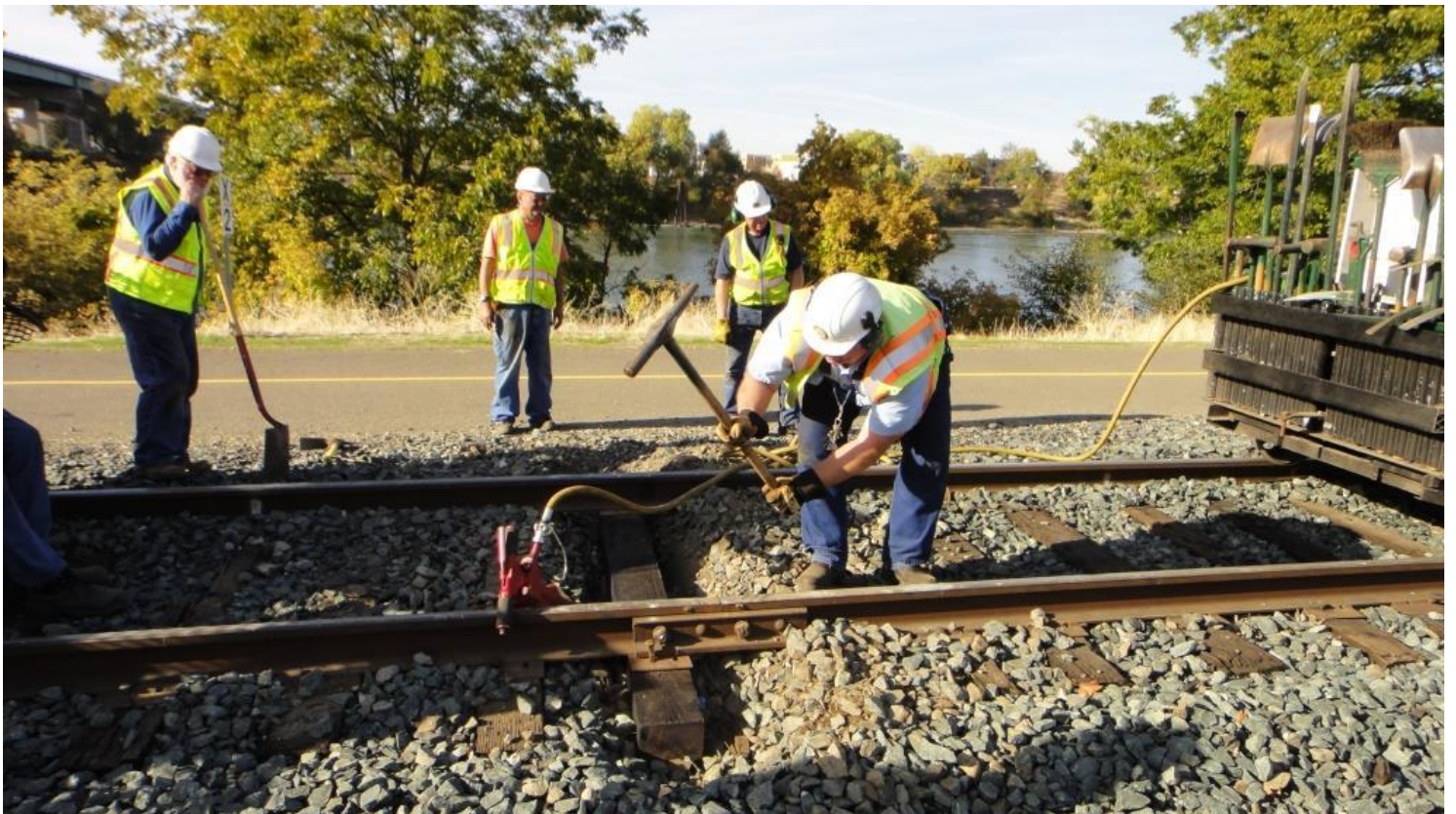
Chris gets in the final word by pounding in the final spike by hand
