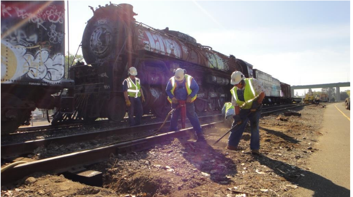
Clem nips the tie while Frank W. uses the pneumatic spiker to drive a spike.
