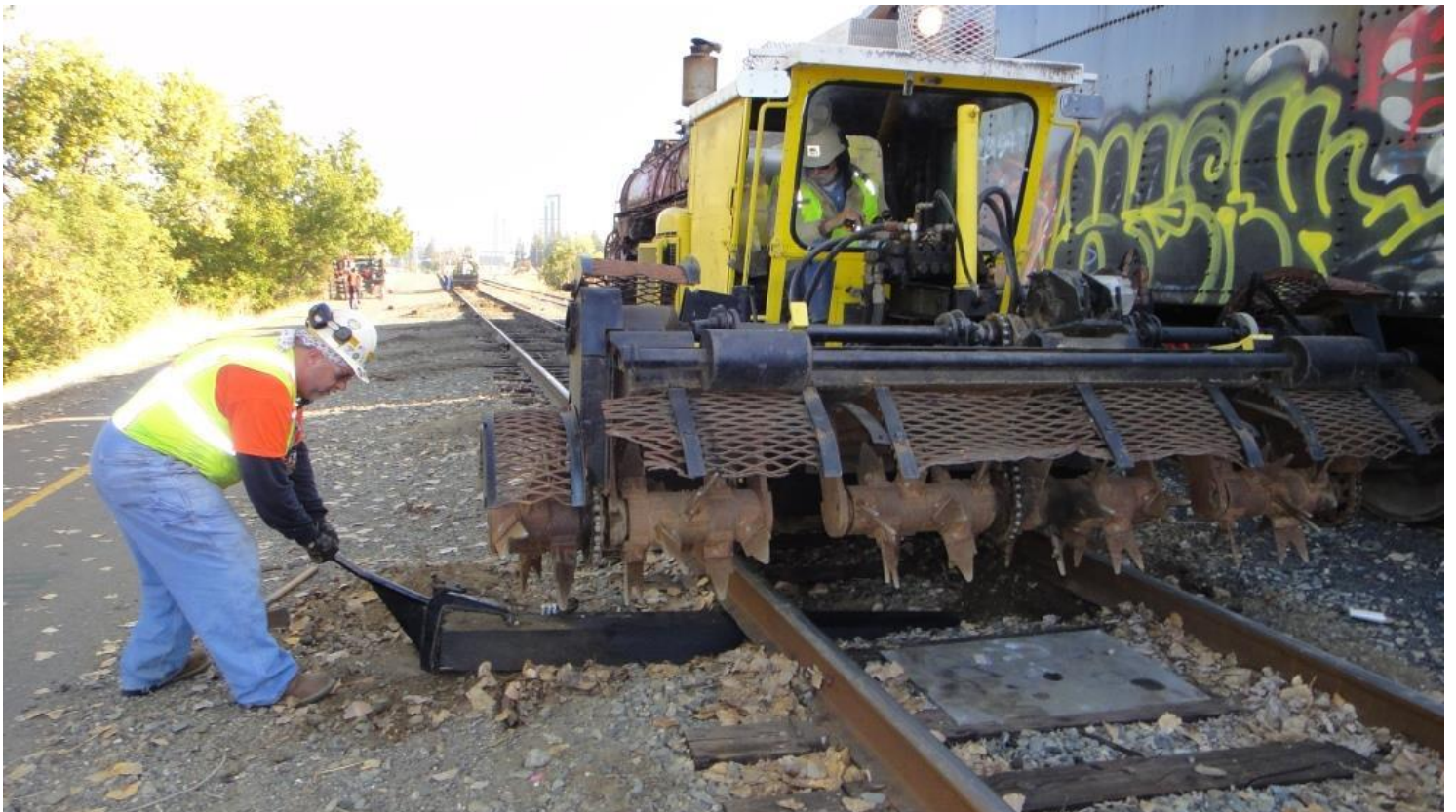
Mike F. guides the placement of a tie that Alan pulls in using the inserter function on the Sacrifer
