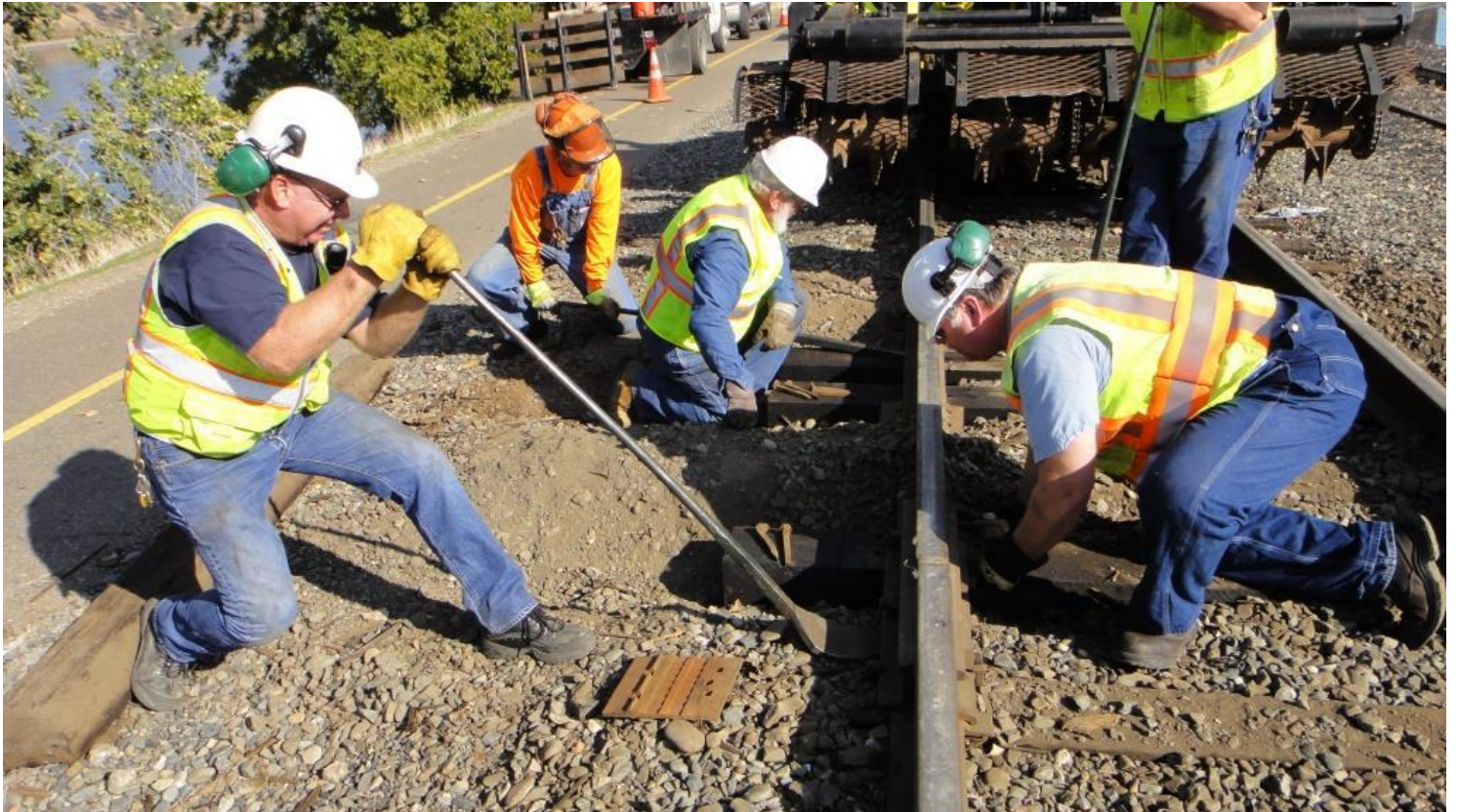
Ed nips the rail while Chris gets a plate under the base
