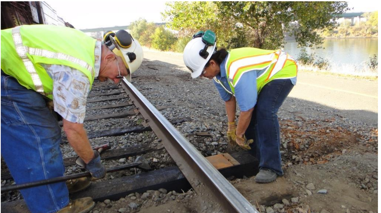
Clem and Pam plate working to get a tie-plate under the base of the rail
