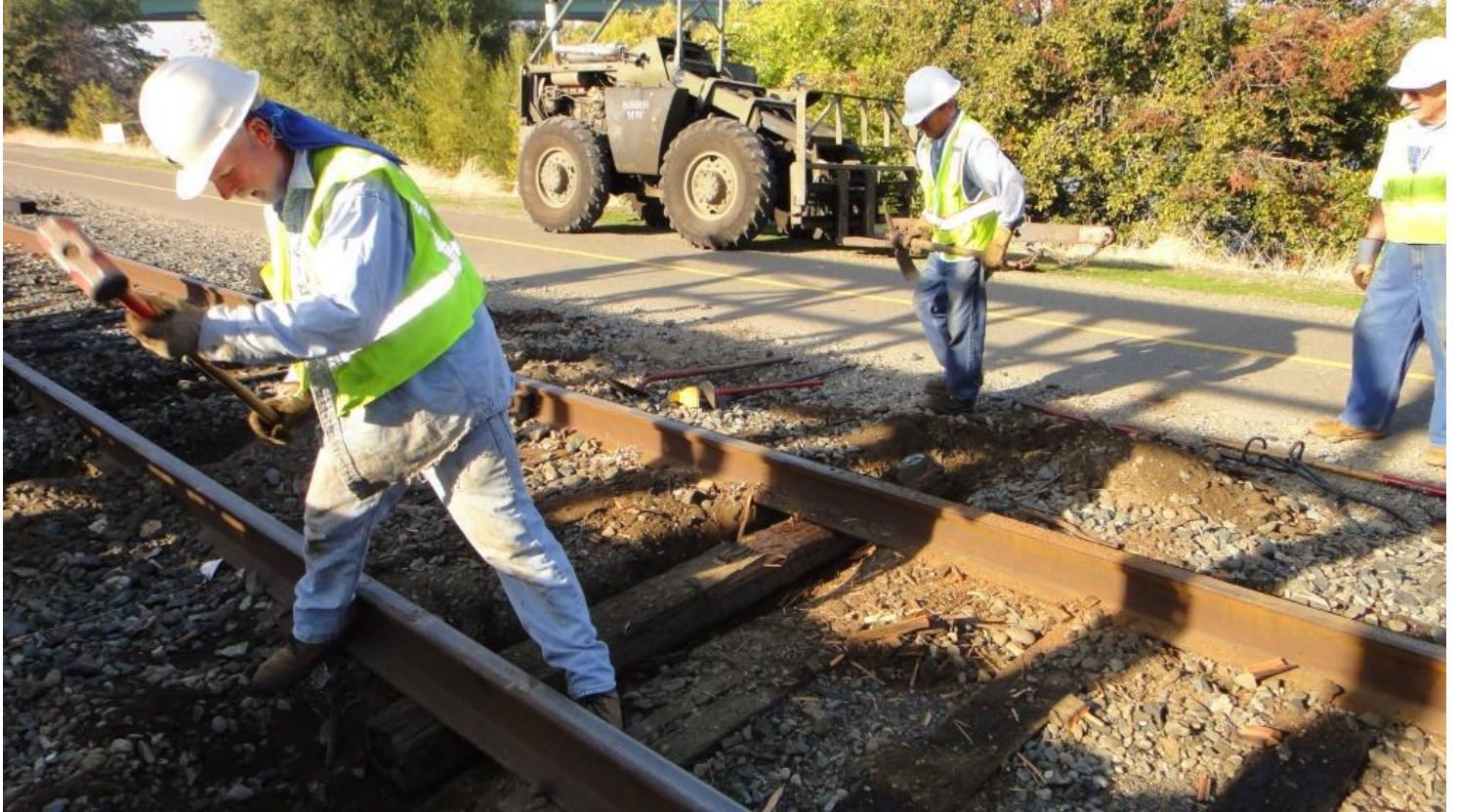
Mike M. and Mike T. team up to dig out a tie
