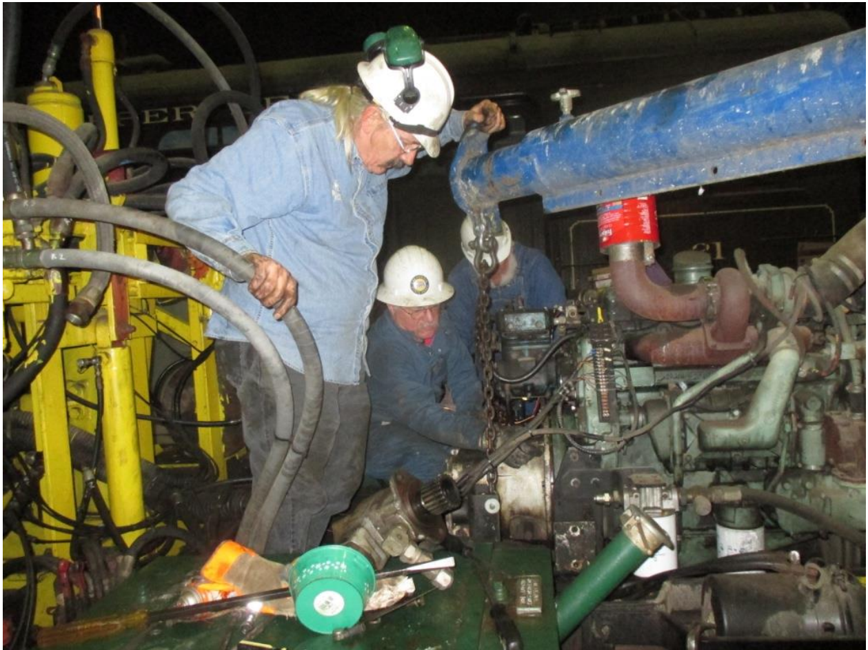
Fred, Mike H., and Frank S. get the Tie-Shear's gearbox reinstalled
