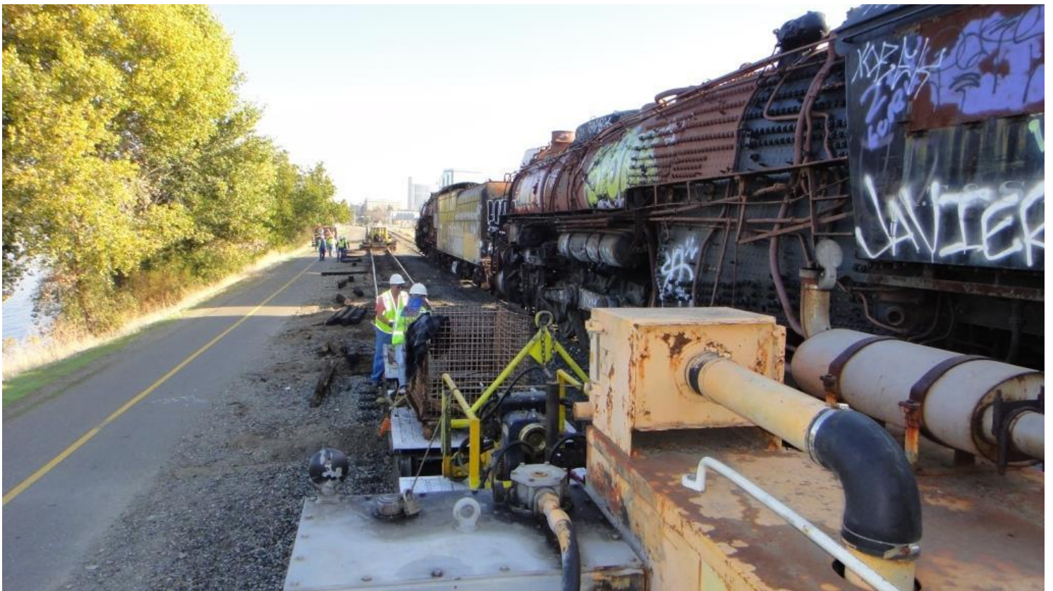
John and Mike M. laying out ties along the line
