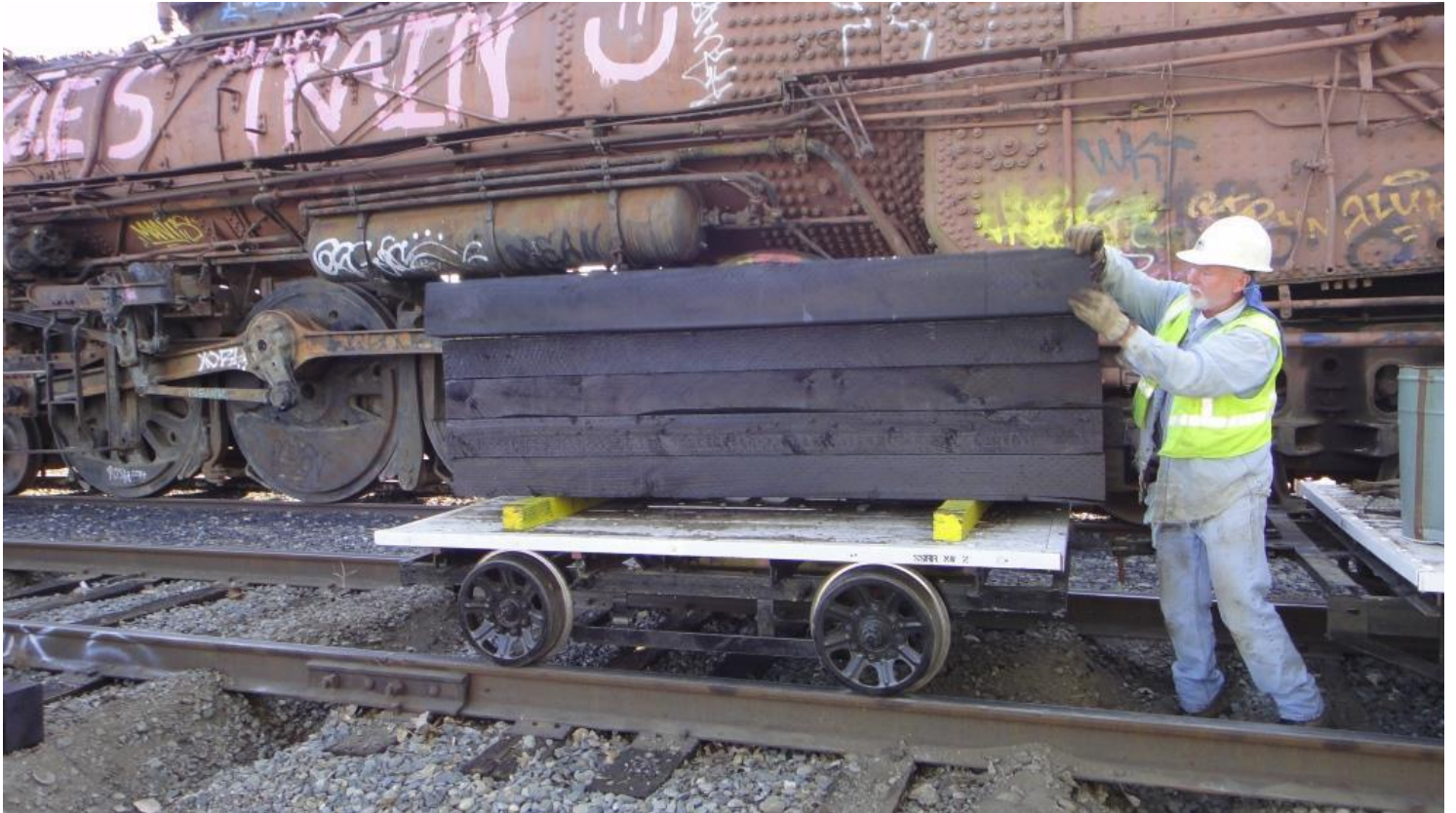
Mike M. rolling a tie off the bundle
